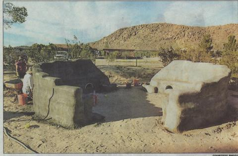
The Sanctuary Project consists of a round earthbag construction that will be lined with ceramic tile. The metal sculpture being made at Bobby Furst's workshop will fill the opposite opening.
